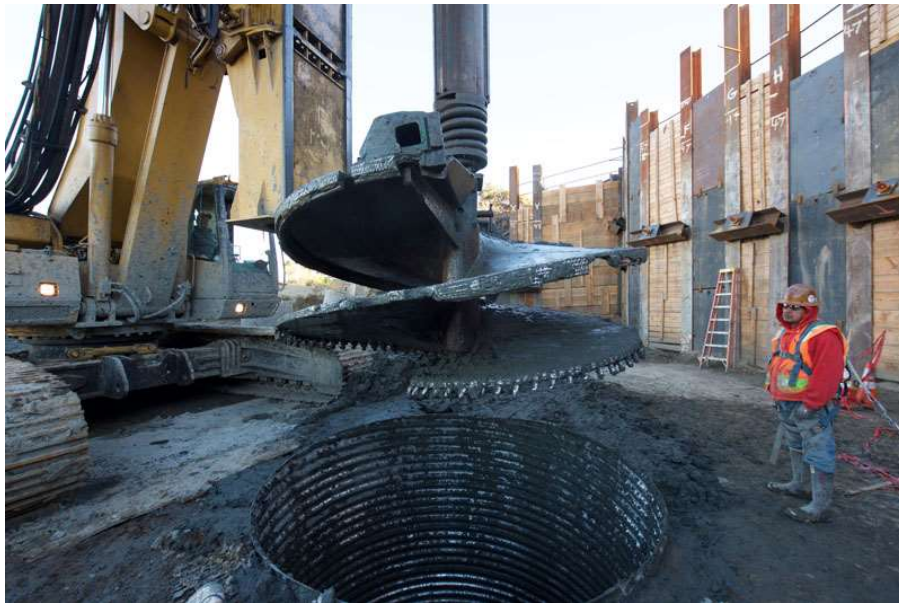
Drilling a footing for a bridge support, December, 2016
